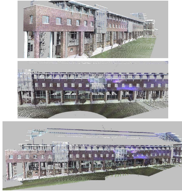
Figure 5. Two scans (top and center) for which range keypoint matching succeeded (bottom), but intensity keypoint matching failed. Range keypoints succeeded despite the highly-repetitive structure of the building since only one correct match was needed.
